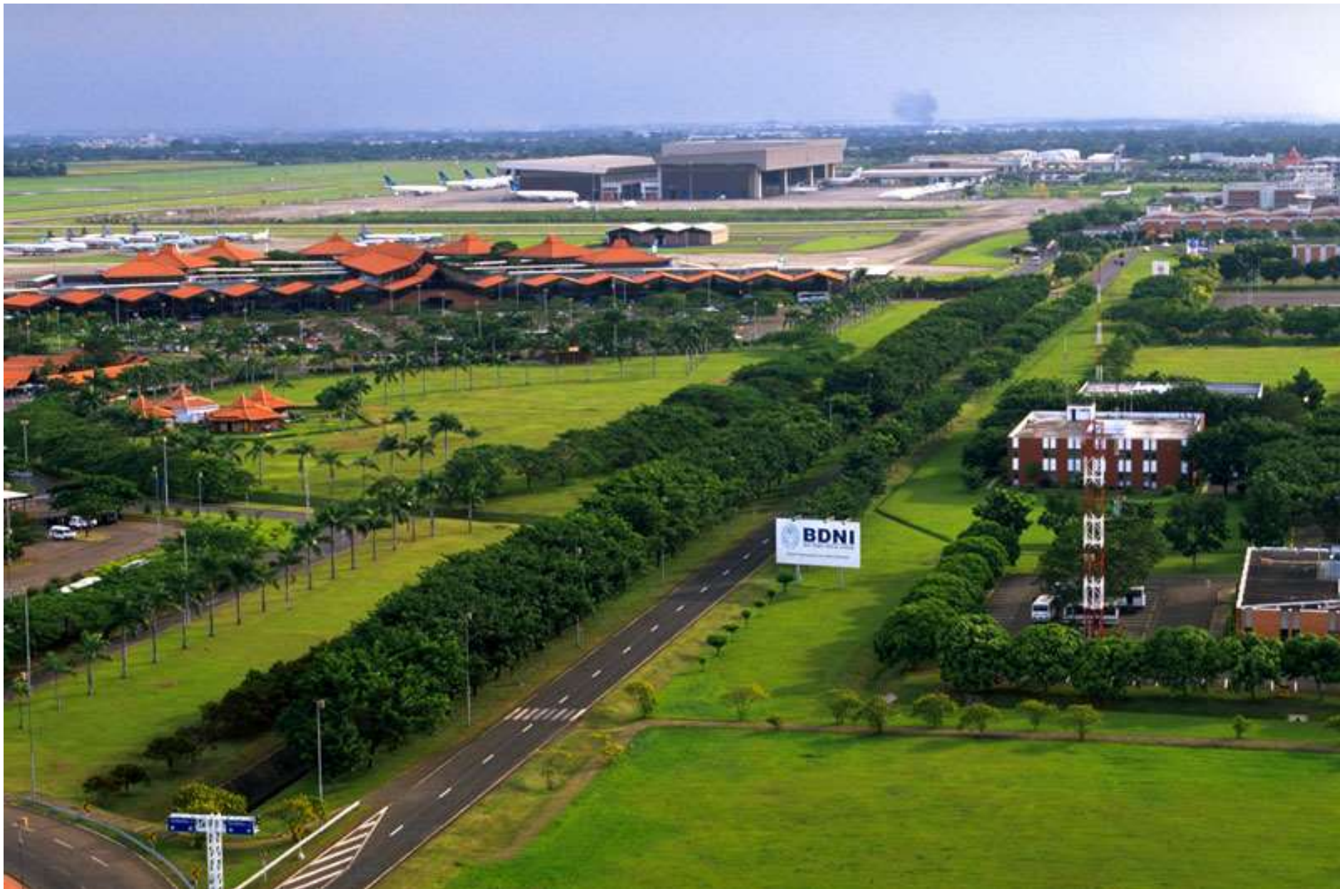
“... integrates landscape and building in an exceptionally beautiful way.” / Aga Khan Award for Architecture, 1995
